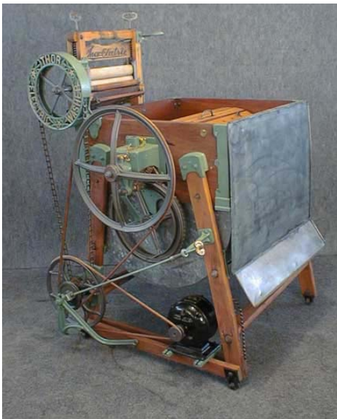
Figure 3. Thor Washing Machine. ca 1911
